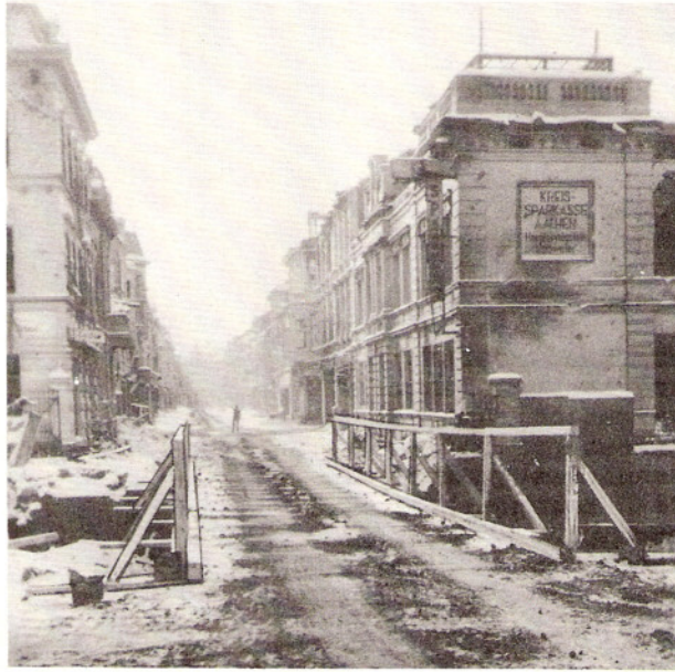
"A" COMPANY'S BRIDGE IN ESCHWEILER, GERMANY. FEBRUARY 1945
