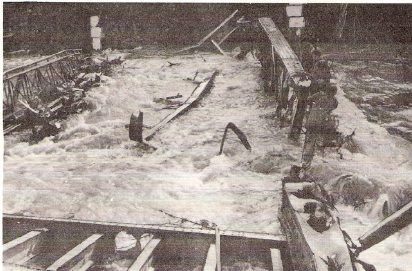
"B" COMPANY'S BRIDGE SITE ON THE INDE RIVER IN ESCHWEILER, GERMANY FEBRUARY 1945
