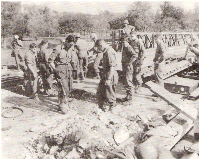
"B" COMPANY WORKING ON THE BRIDGE APPROACHES BETWEEN GULPEN AND VALKENBURG, HOLLAND. SEPTEMBER 1944
