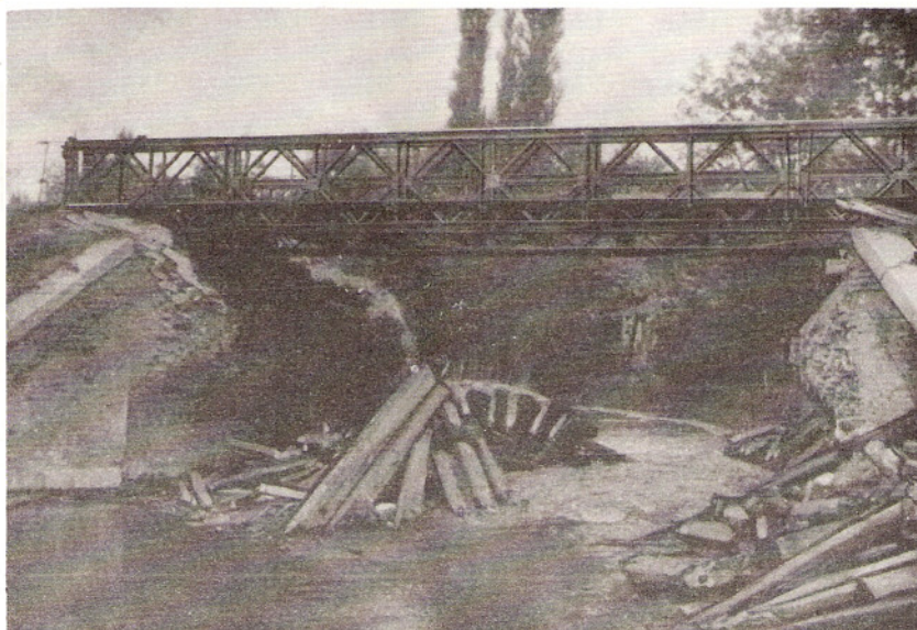
"C" COMPANY'S BAILEY BRIDGE EAST OF GULPEN, HOLLAND. SEPTEMBER 1944
